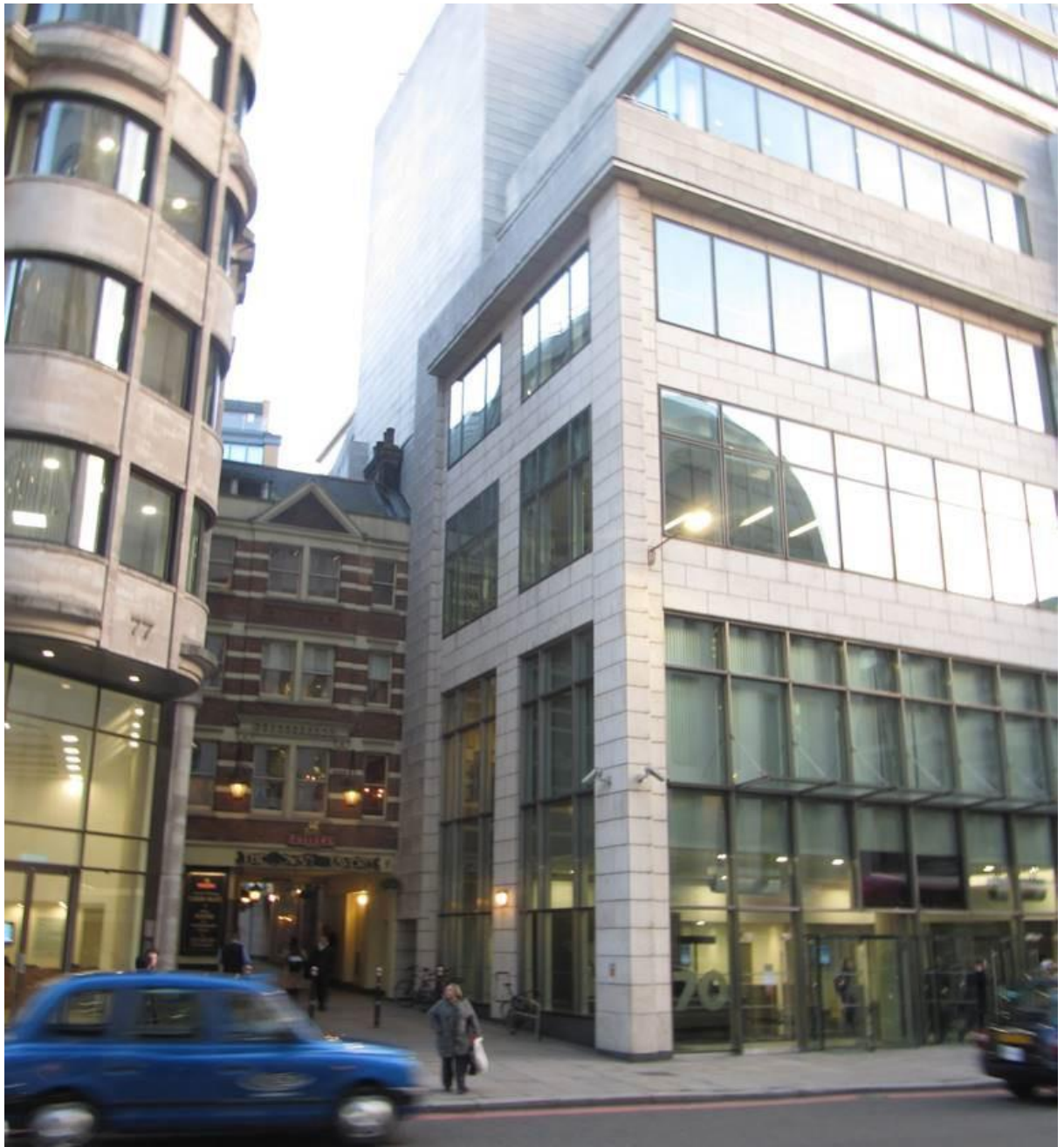
Image 4: View of existing building at Ship Taverns Passage
